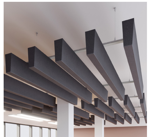
5 BEAMS VIGA (D401) IN SLATE (P105)
